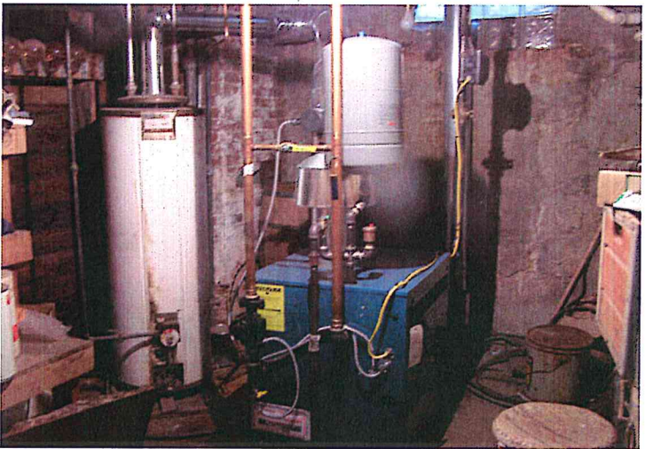
Basement utility area
