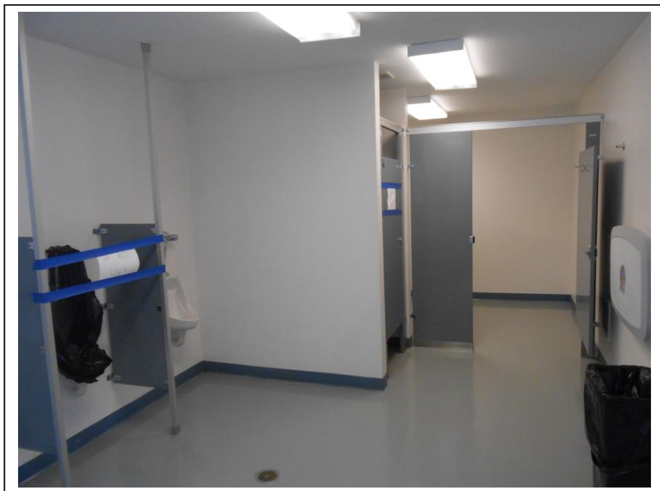
Typical Restroom View
