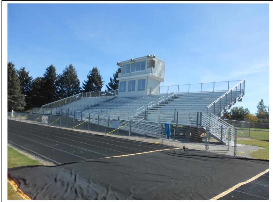
View of Southern Bleachers w/ Press Boxes facing southeast
