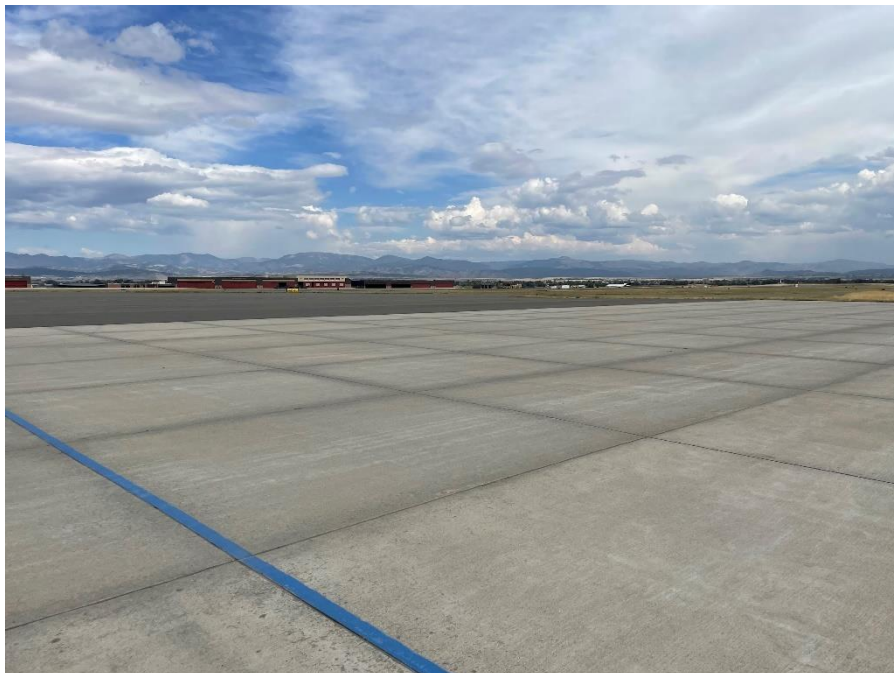
Concrete paving, aircraft parking, and access to the tarmac
