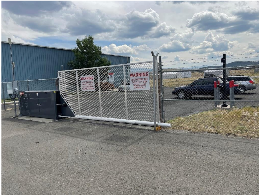
Secured access gate
