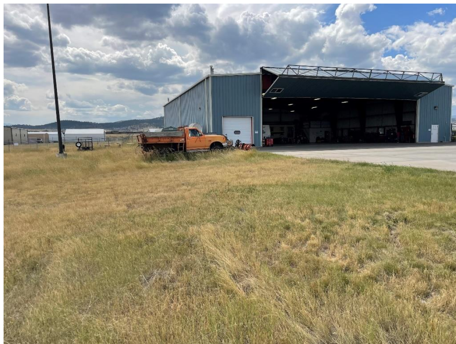
Airport access – Schweiss electric bifold door
