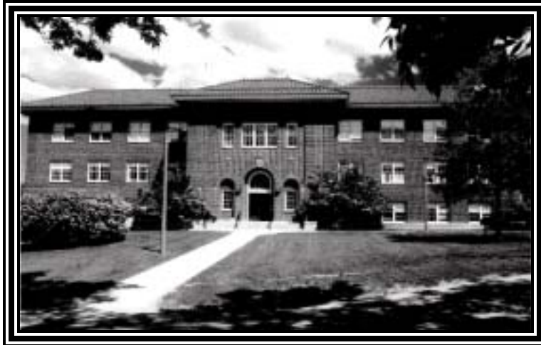
Herrick Hall – Constructed 1926 Health and Human Development Department Gross Area 40,400 s.f.
