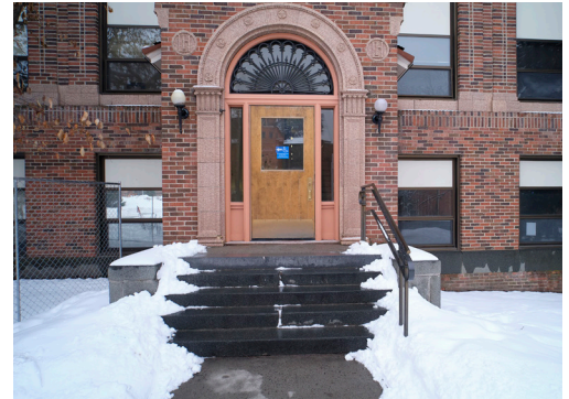
Lewis Hall is inaccessible under the ADA.
