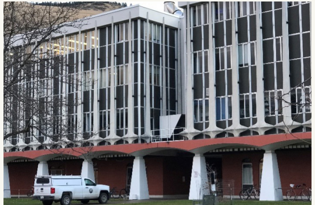
Clapp exterior view
